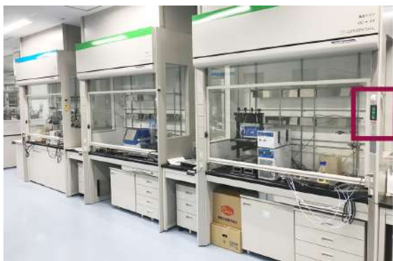
Low air volume (push/pull type), ultrahigh speed variable air volume (VAV) local ventilation device (exhaust fan output visualized on the operation panel) (Minase Research Institute)
